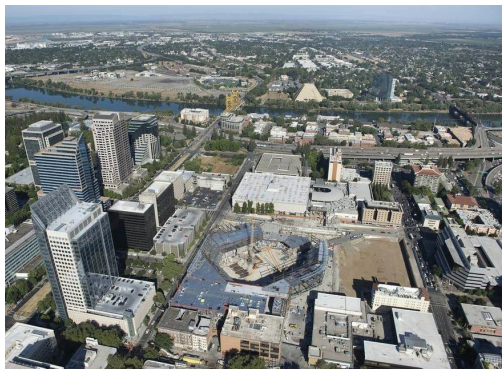
The downtown arena under construction on Friday, June 12, 2015 in Sacramento, Calif. (Randy Pench rpench@sacbee.com)
